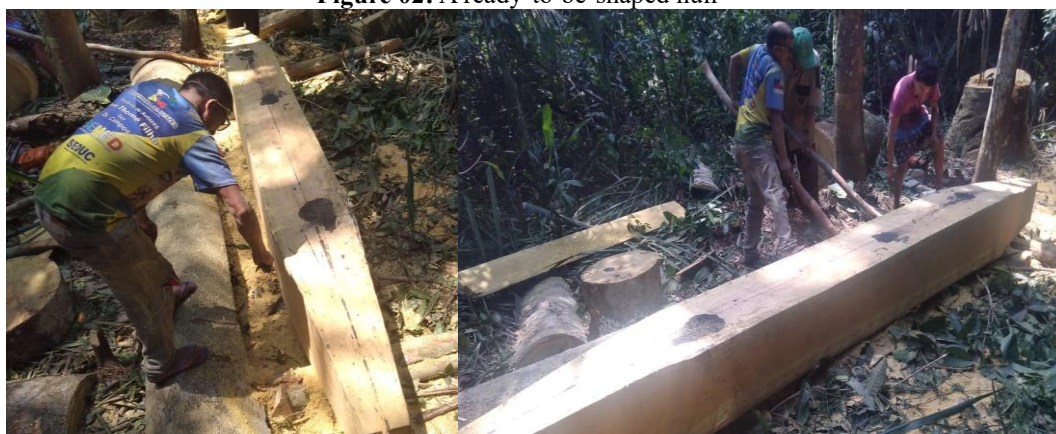
Figure 02: A ready-to-be-shaped hull
